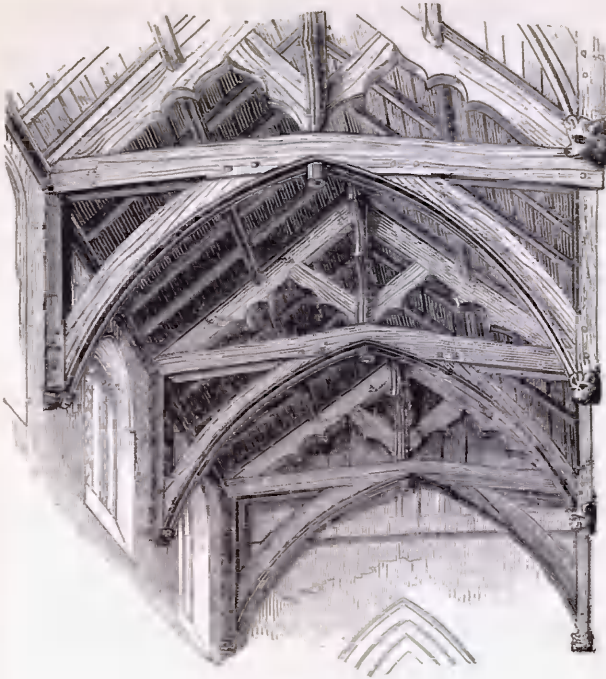
Roof, west end of Nave.
